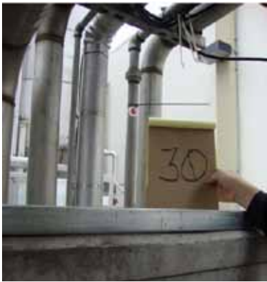
Leaks Identified & Repaired
